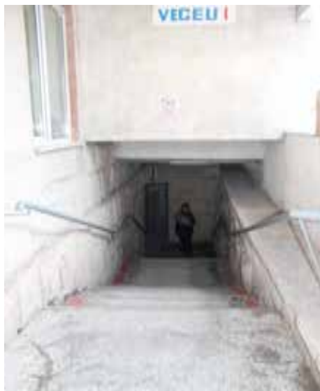
Public WC at the South bus station
